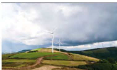
Glenough Windfarm Irland, County Tipperary
