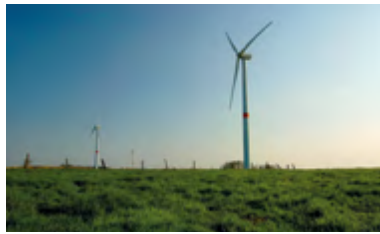
Windpark Losheim Saarland
